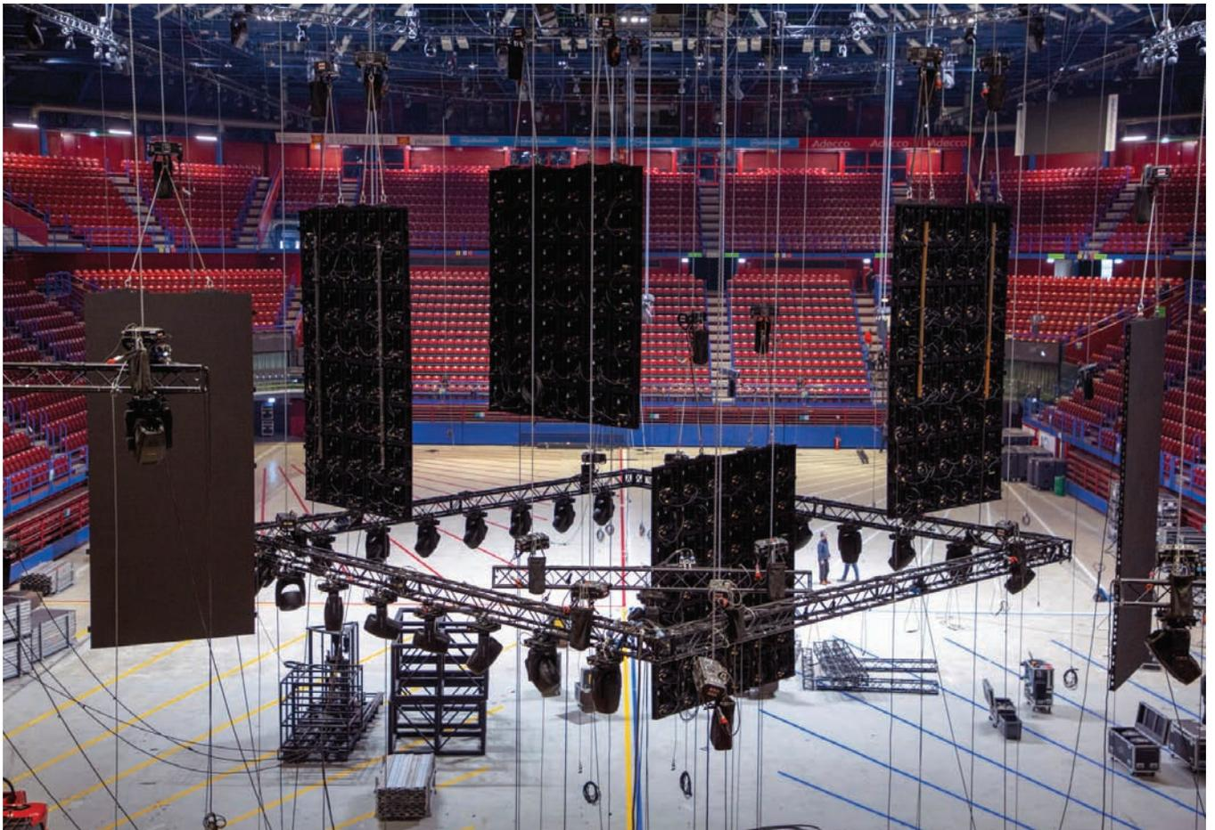
EXE Rise and Litec truss, the lifting of the centre ceiling.
